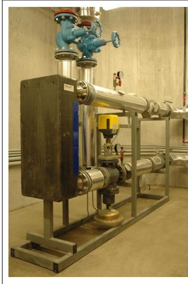
Example installed heat exchanger in a mechanical room
