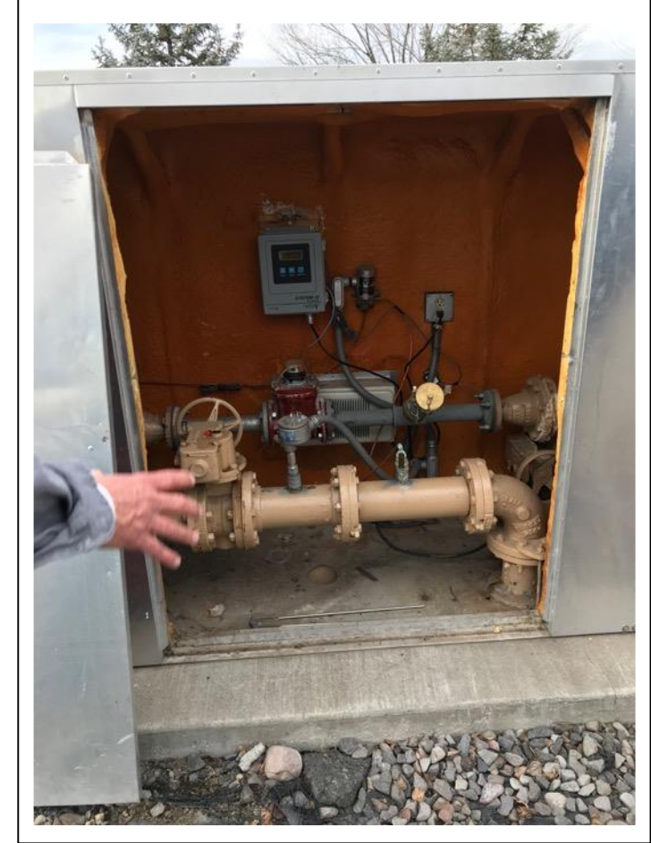
Example heat exchanger building enclosure outside → Used if no room inside building
