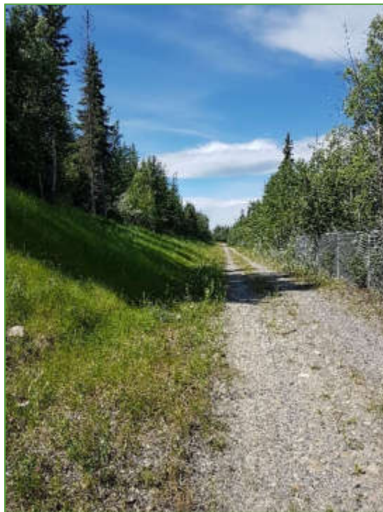
Figure 51 - Photo of Narrow Service Road with Steep Side Slopes along proposed ROW
