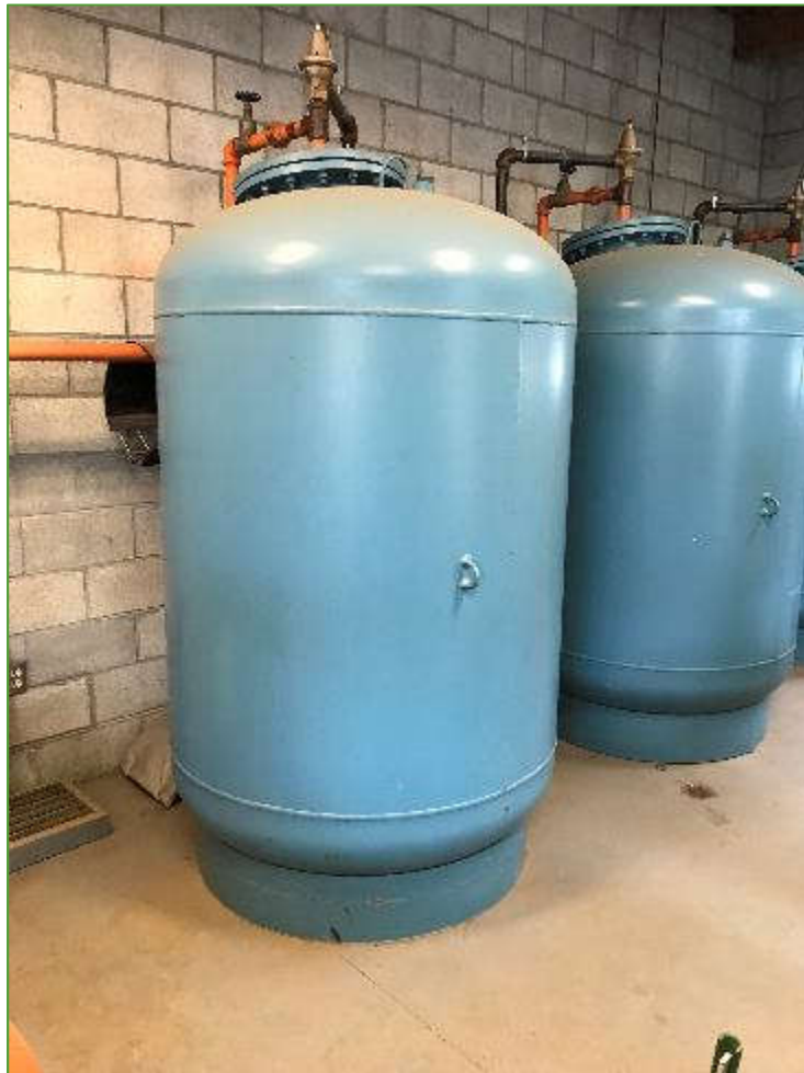
Figure 61 - Expansion Tank Configuration - Klamath Falls, OR
