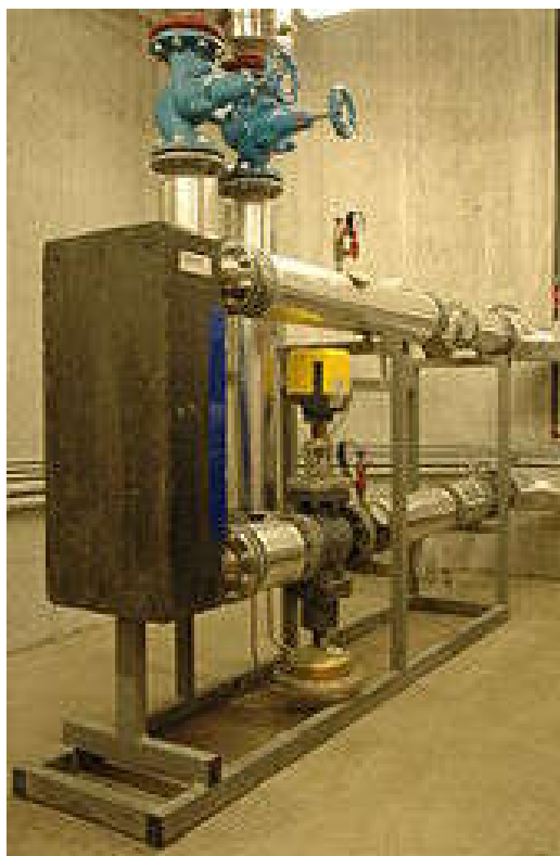
Figure 76 - Photo of Installed Heat Exchanger in a Mechanical Room [66]
