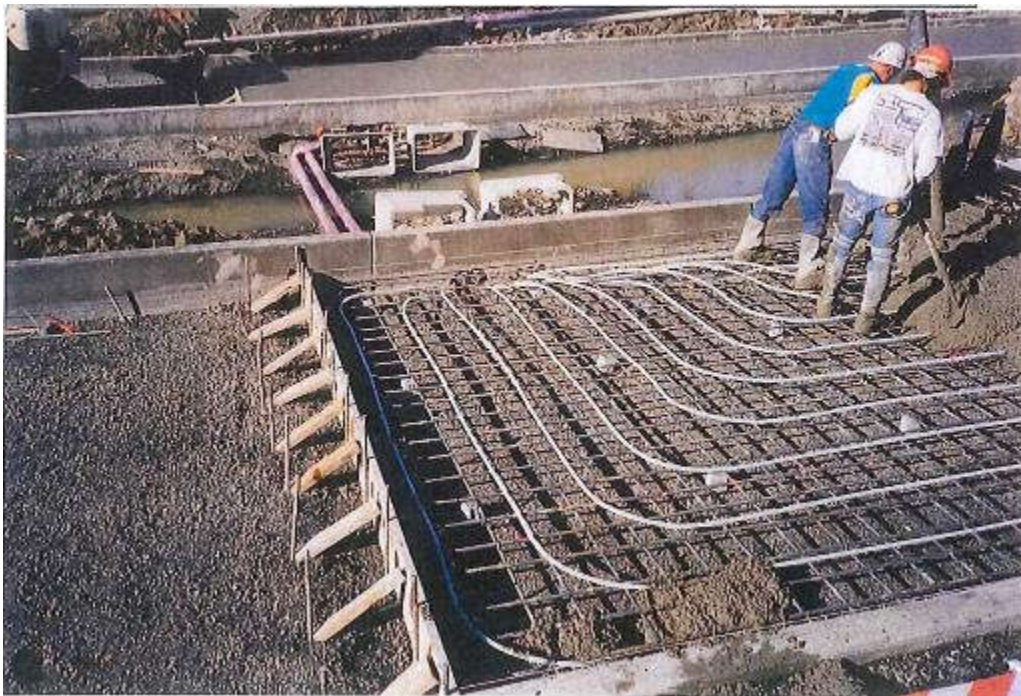
Figure 44 - Example installation of a hydronic snow melting system
