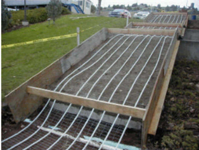
Figure 42 - Example Snow Melt System - Stair Construction, Klamath Falls, Oregon [37]
