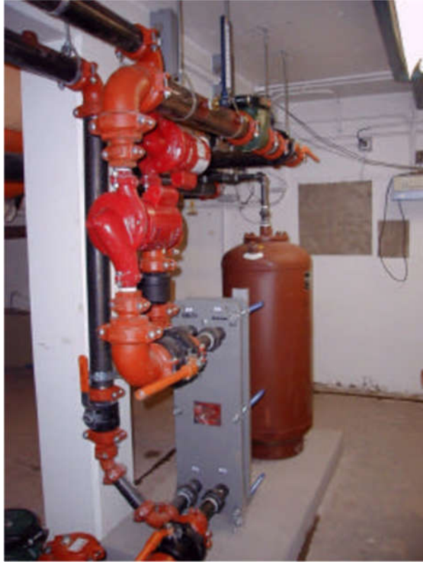
Figure 41 - Example Back End of Snow Melt System, Klamath Falls, Oregon [37]
