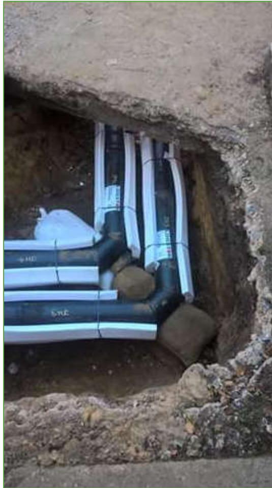
Figure 48 - Example Foam Pad Installation for Logstor Pipe System [46]
